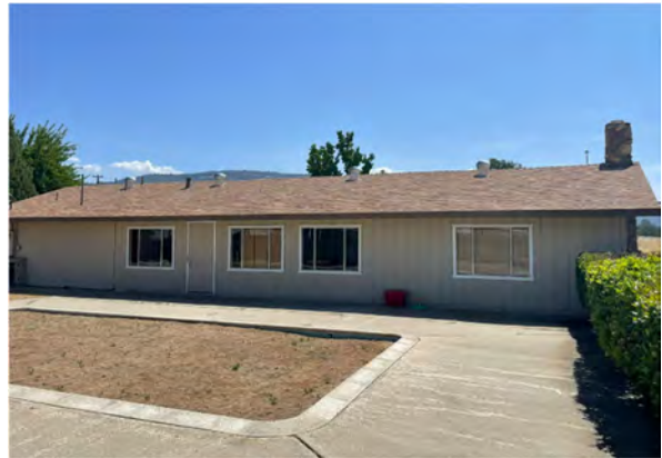
Rear of Clubhouse
